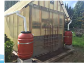
Our Rain Collection System
